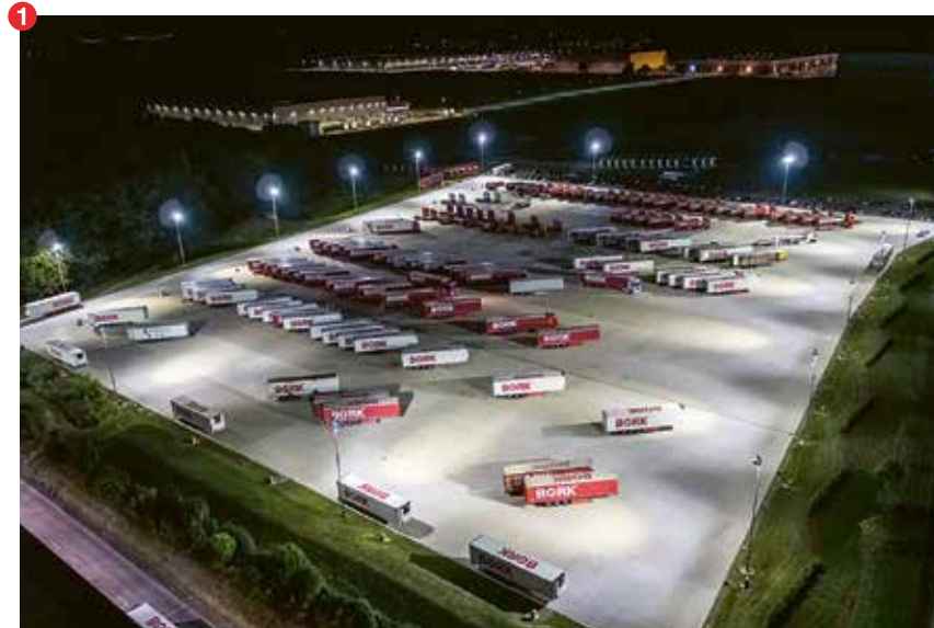
Project: Bork, Langgöns Product: Floodlight FL 20
